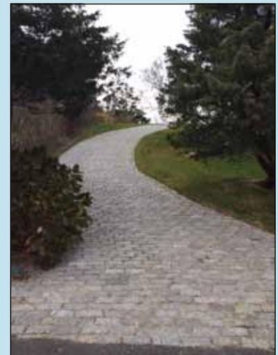
An example of permeable paving in Tisbury, a gently sloping driveway with pavers that allow runoff to fall between them.
