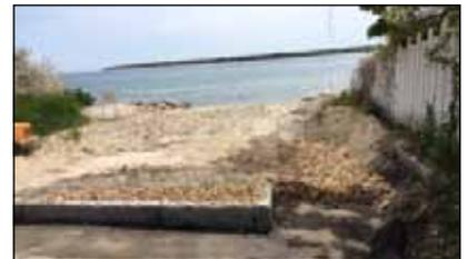
Since our get together, the DPW has been working at Grove Avenue (photo) installing a granite barrier at the end, building up the sand supply behind it and creating a gravel-filled passage at an opening just to the right of the barrier to help filter off stormwater runoff. The project will also reduce the volume of water cascading down Grove before it reaches the harbor. Similar work will be done at the public access off of Hines Point. We appreciate these speedy first steps.
